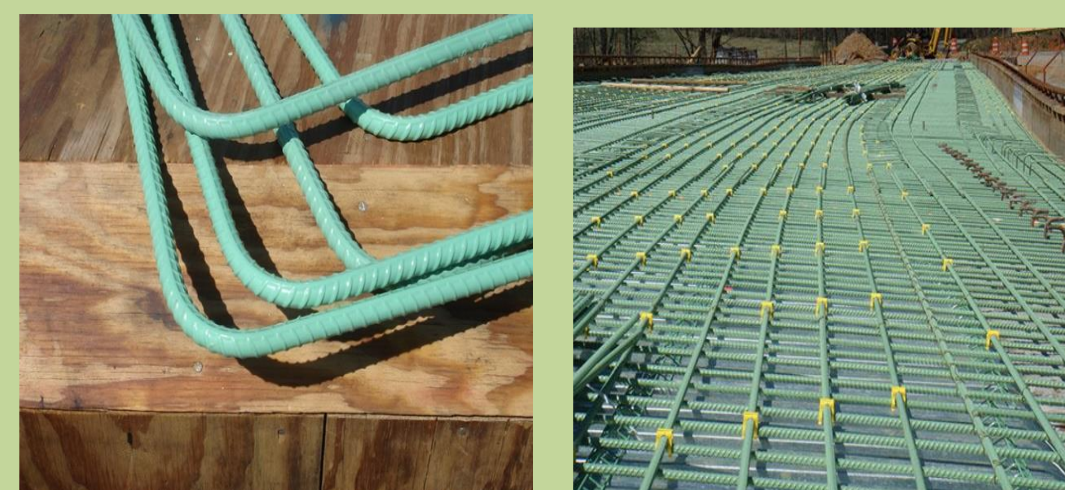
Figure-3 a) 90 degree bent with epoxy coated rebars. b) mesh of epoxy rebars in a bridge deck.
